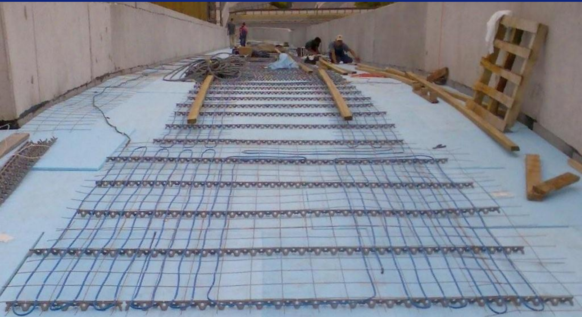
Solvay Park Shopping Centre, Cracow, Poland ramp heating, 570m lanes
